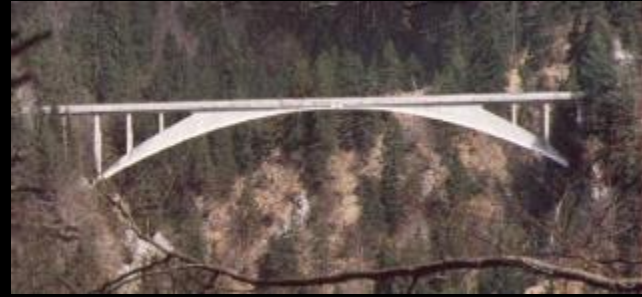
Salginatobel Bridge Schiers, Switzerland Robert Maillart 1930
